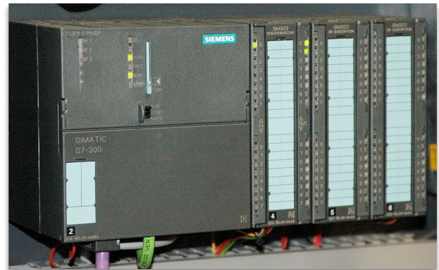
Siemens Simatic PLC
